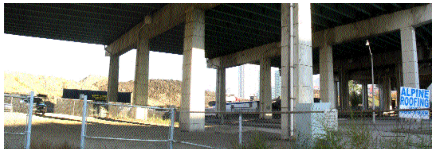
View of the Gardiner Expressway, looking northeast, towards the Golf Course on the Railway Lands Neighbourhood
