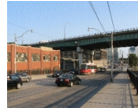
Bathurst Street, looking south
