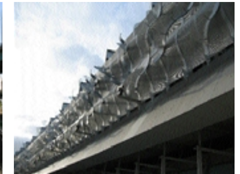
Entrecampos Railway bridge, Lisbon
