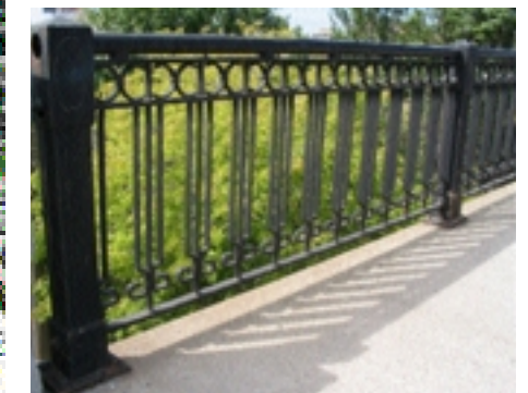
The existing railing should be kept or used locally.
