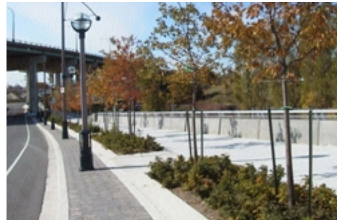
Fort York Boulevard, close to Bathurst Street, looking west
