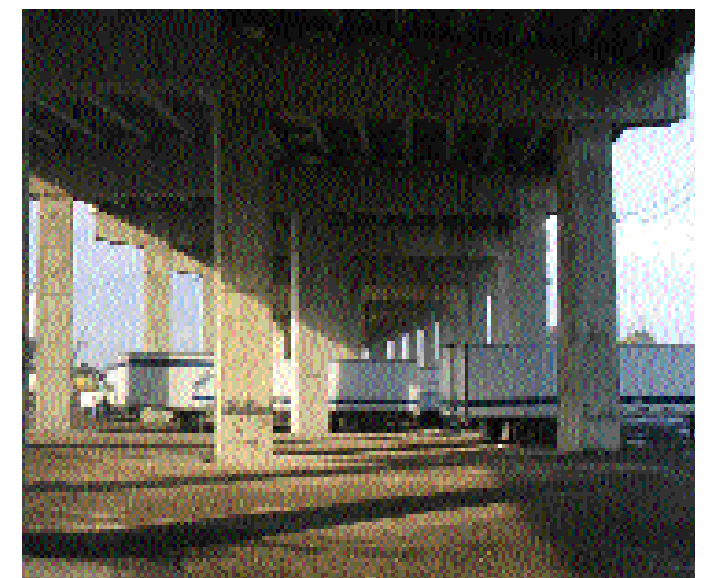
View of the Gardiner from Bathurst Street, looking west
