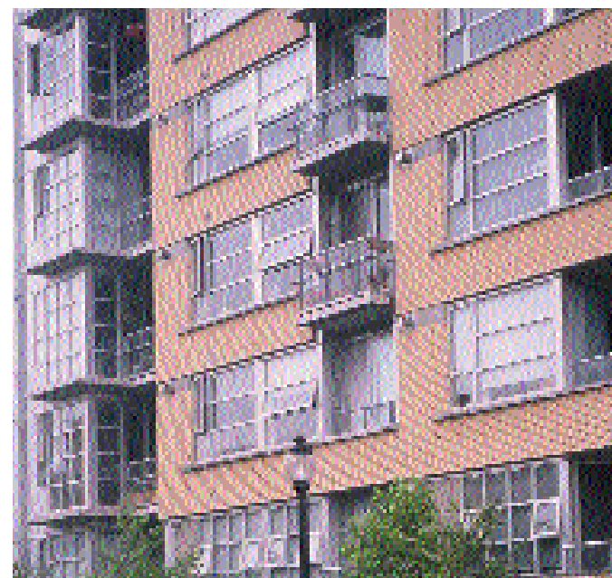
Balconies integral to the building - Arbutus Industrial Lands, Vancouver
