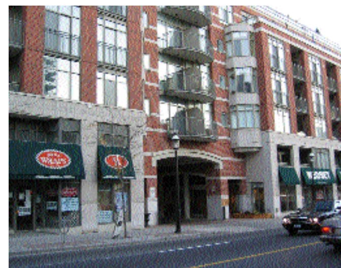
Parking and service entrance – Jarvis Street, Toronto
