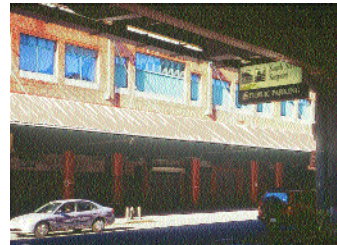
Loading frontage, South Street Seaport, New York
