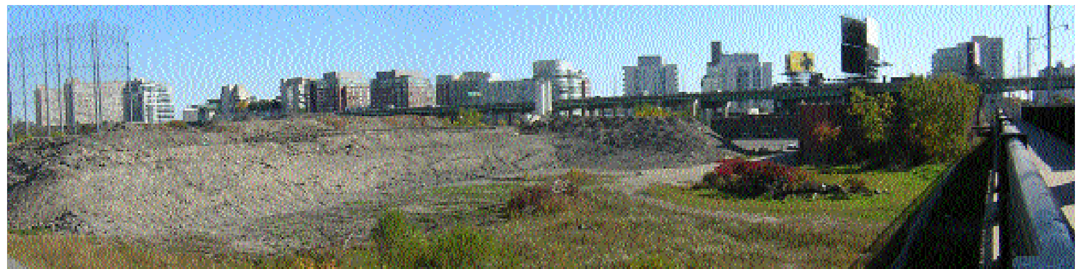
View of the area of the park, showing the fill in place for Bremner Boulevard, looking southeast
